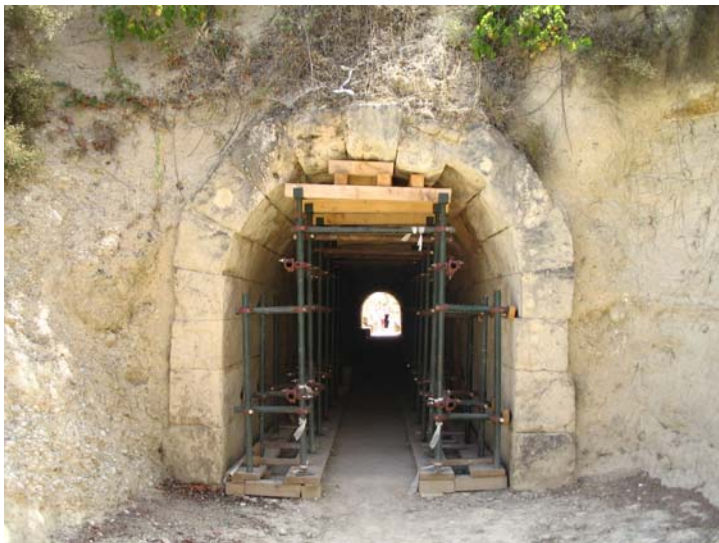
Tunnel from the West, 2007, with Emergency Scaffolding in Place
