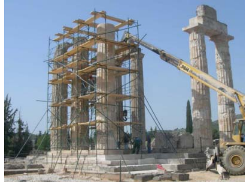
Crane donated by Titan in use erecting column. (Source: Makris Report on Reconstruction 2007)
