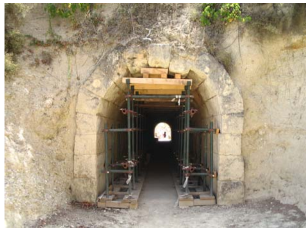
Stadium Tunnel With Bracing Scaffolding
