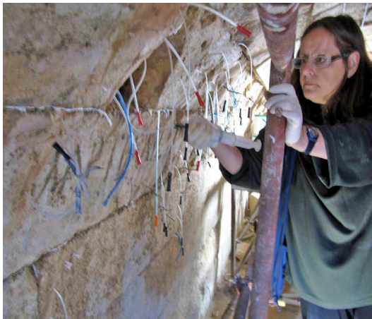
The head of the conservation team, Ioanna Dogani, inserting grout with a syringe.
